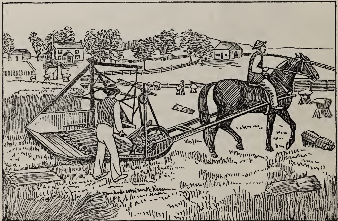
FIG. 42.—McCormick's reaping machine (1834).
